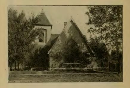
Church at Osage City, Kansas. An attractive and commodious building seating about 300 in the main room. The chapel, which can be opened into the larger room, will accommodate about 100. Built in brick or stone it will cost from \$4,500 to \$5,500. For ground plan see next page.
